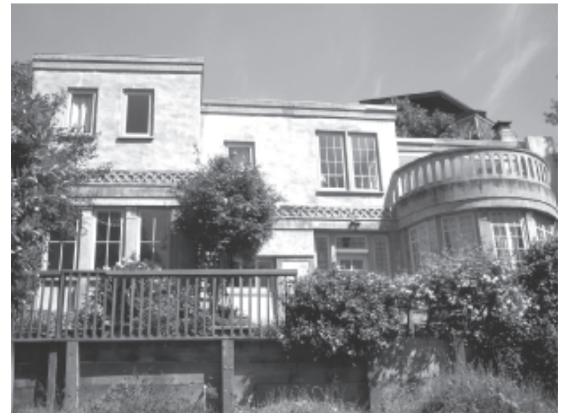
Figure 10: Christopher Alexander, Upham House (1992): A very appealing building, but the decorative detailing seems to deliberately avoid historical styles, as if he wanted to design a classical balustrade and cornice but did not dare. (Photograph by Charles Siegel.)
