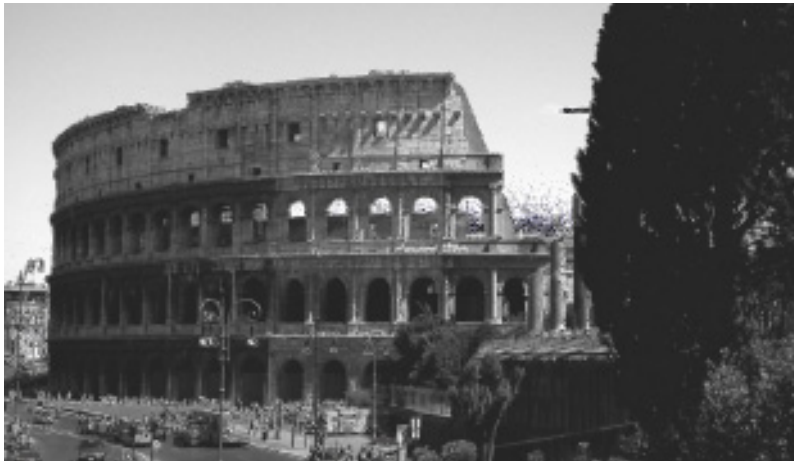
Figure 5: Colosseum (80 AD): The structure is made of three levels of arches topped by a wall. Columns in three orders are placed in front of the arches, and pilasters are placed in front of the wall, as decoration with no structural function. (Photograph by Dafialis.)
